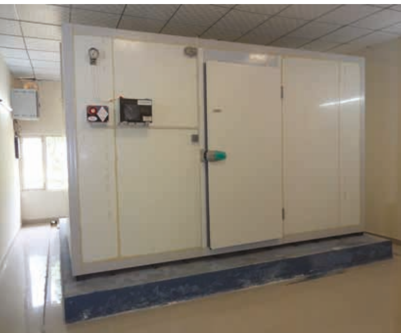
Model WIC / WIF installation at NCCVMRC
